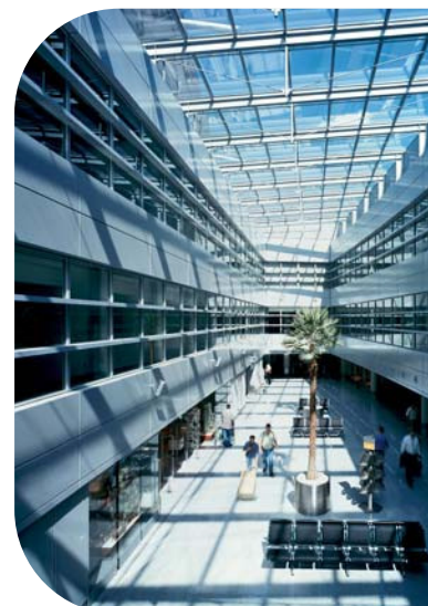
Partition with Pilkington Pyrodur ® – International Airport, Düsseldorf (D).
